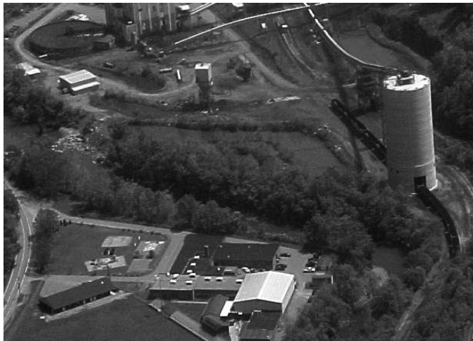
The current (soon-to-be former) Marsh Fork Elementary sits within 300 feet from one coal silo and 400 yards from a leaking sludge dam. (Photo by Brittany Williams).
