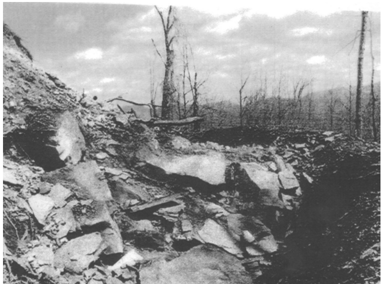
From the OSM report sent to Bo Webb after the investigation: documentation of Massey's failure to control sediment ditches.
